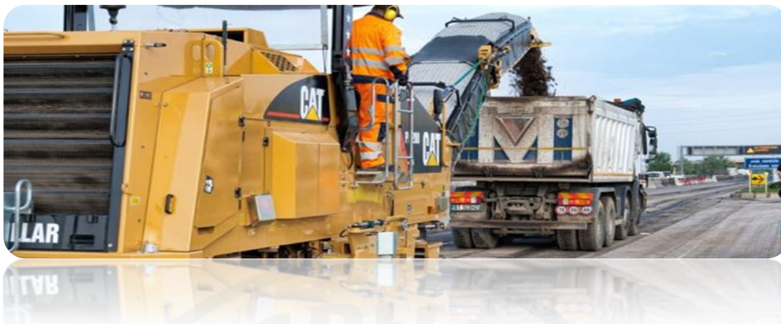
Figure 25. Example of cold recycling treatment.
